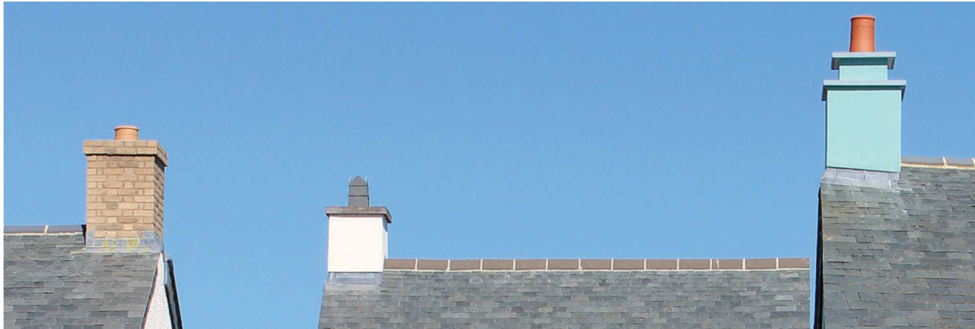
Traditional brick chimney with clay pot; rendered chimney with slate pot and rendered chimney with clay pot
