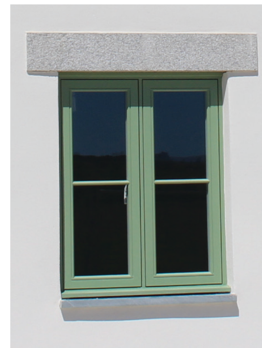
Side hung casement, granite lintel and slate cill.
