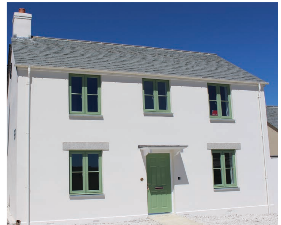
Granite is used for lintels and landscaping. Slate is used for cills and roofs.
