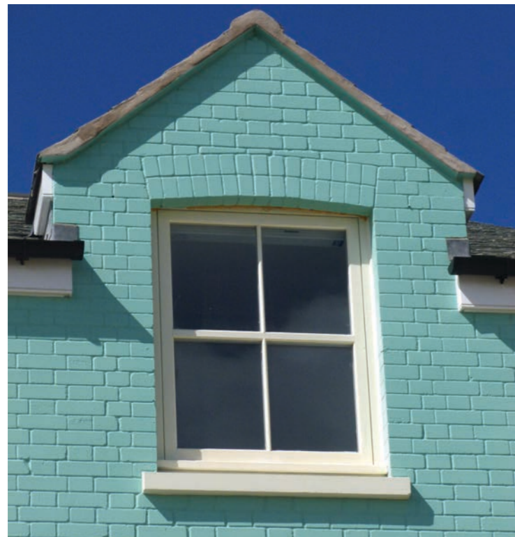
Good example of a half dormer with clipped eaves
