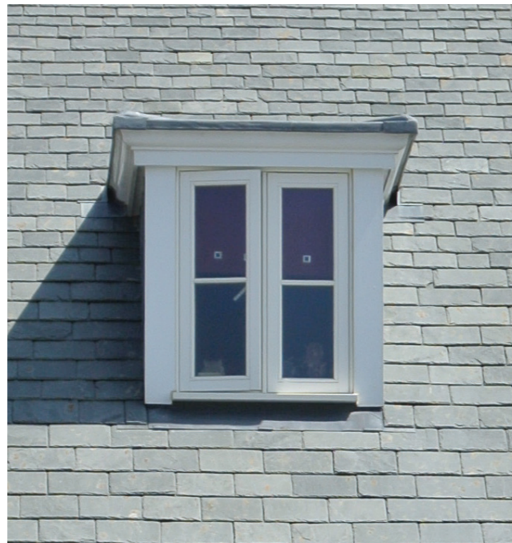
Good example of dormer window with cornice
