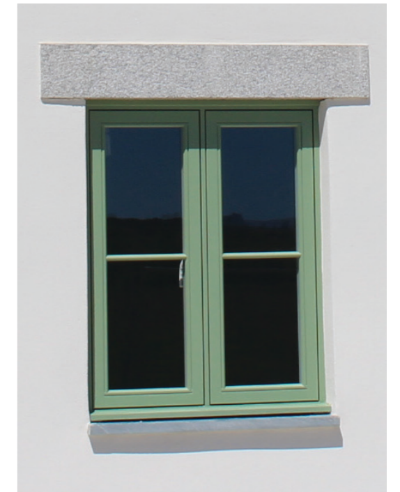
Side hung casement, granite lintel and slate cill.
