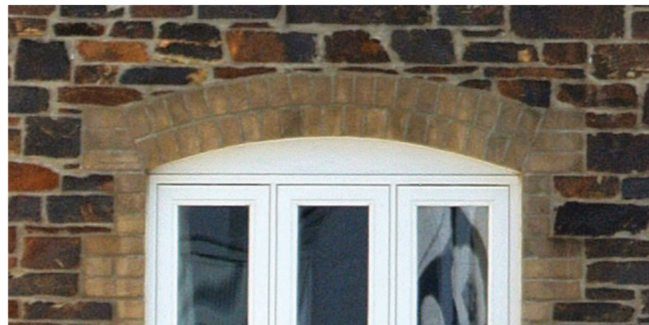
Segmented brick arch
