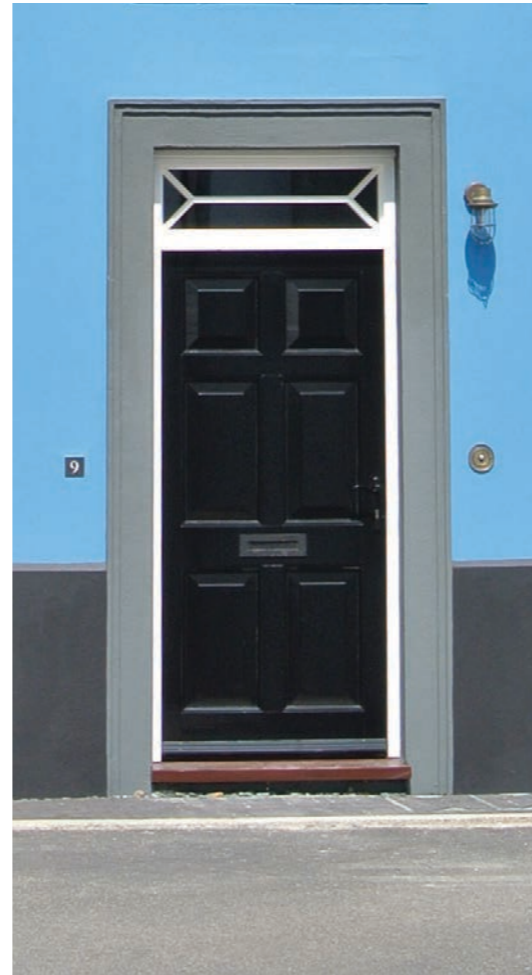
A well-proportioned six panel door with lights above.
