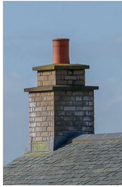
Traditional brick chimneys with clay pots and a rendered chimney with slate pot
