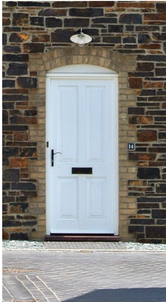
A simple door with rough brick arch and quoins.
