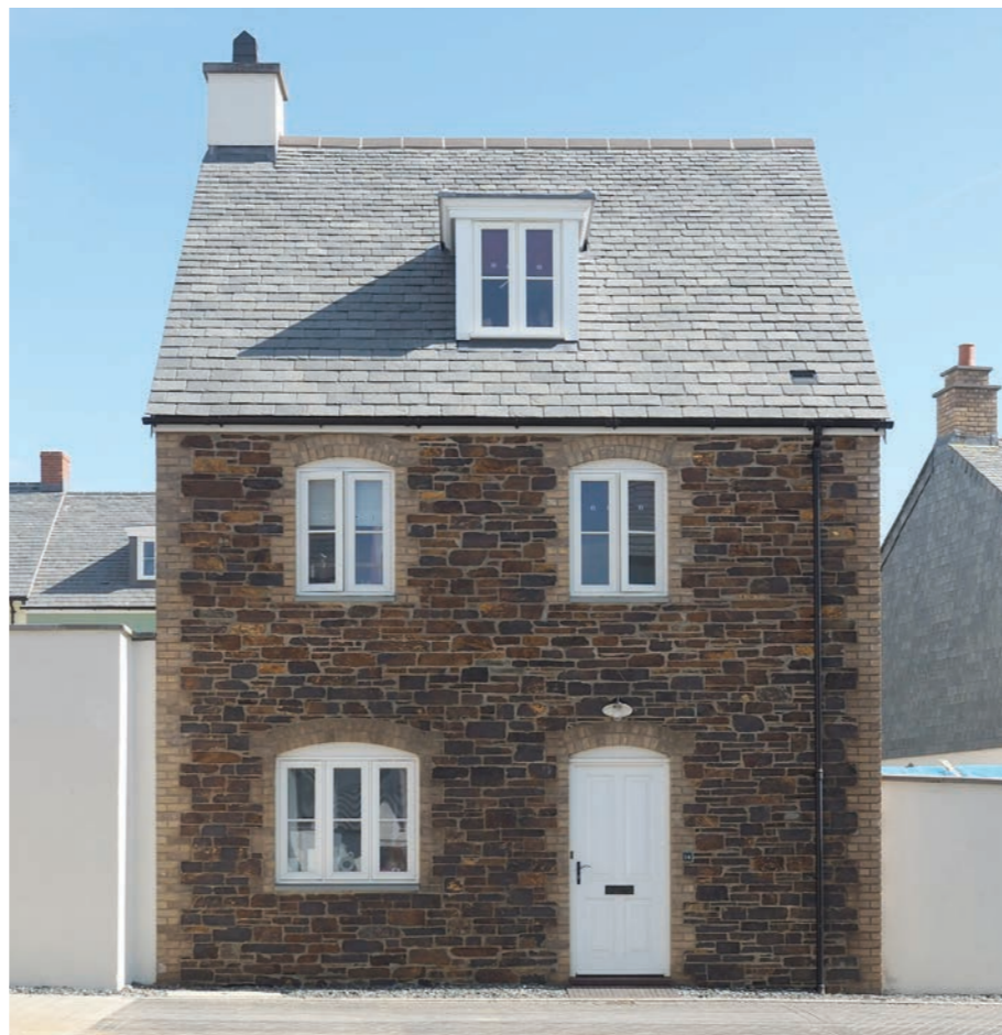
Yennadon stone with brick quoins
