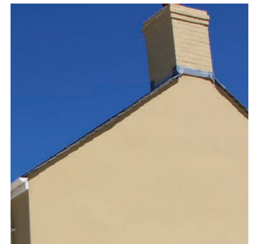
Simple Verge with wall finish taken up to underside of roof
