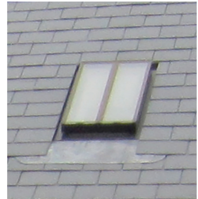
Conservation type of rooflight flush with the roof
