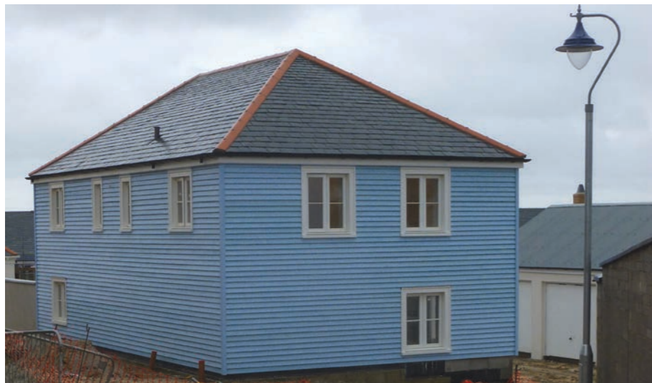
Painted timber building
