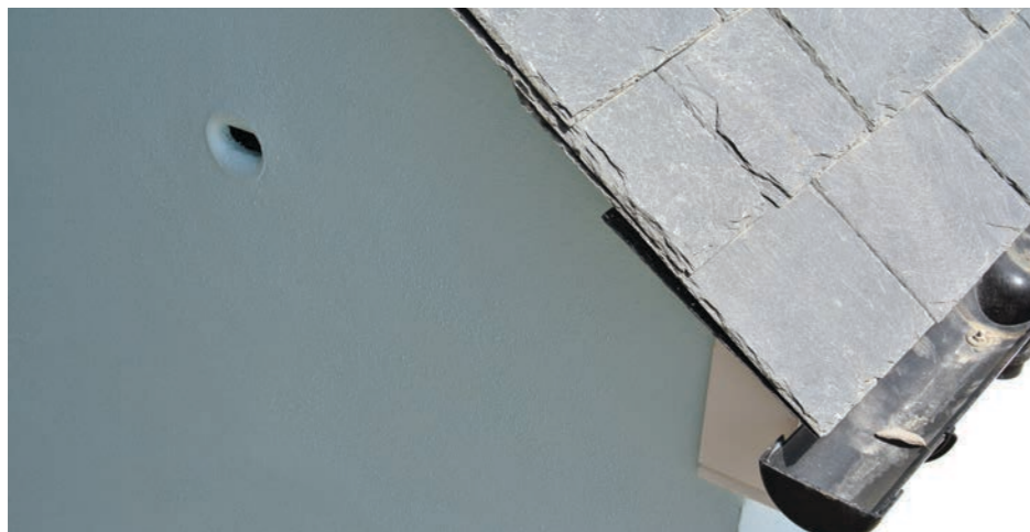
Close Clipped eaves
