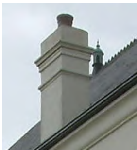
Traditional slate pot on chimney
