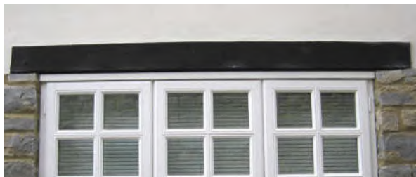
Hardwood timber lintel
