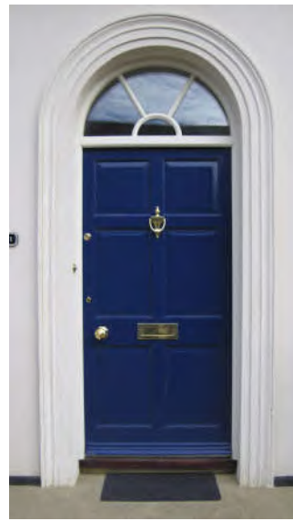
Good examples of well proportioned doors and lights above. Authentically detailed six panel type doors. The upper panels may be glazed
