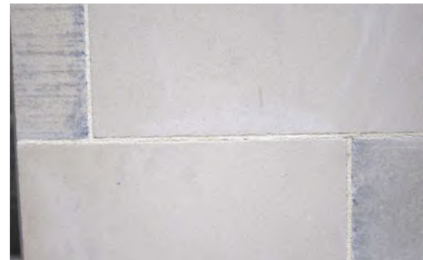
High quality Ashlar with tight mortar joints
