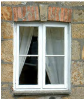
Side-hung casement window & slate cill
