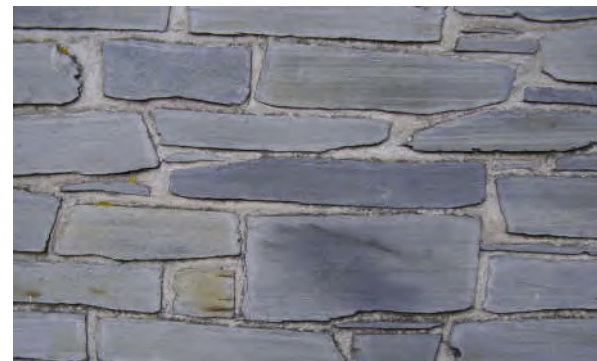
High quality sawn stone wall with appropriate mortar colour and pointing profile to reveal full colour and texture of the stone
