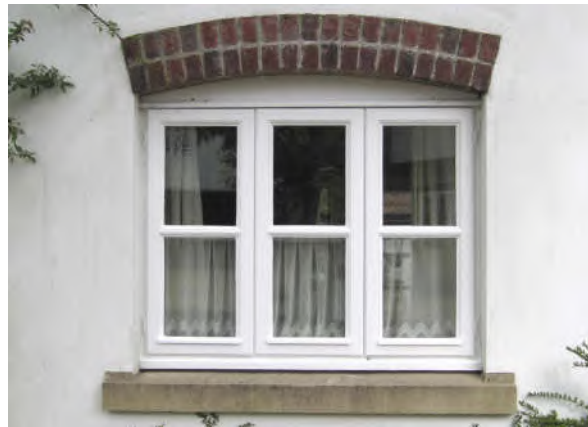
Side hung casement, brick arch and stone cill
