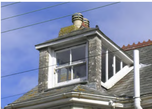
Dormer with glazed side panels
