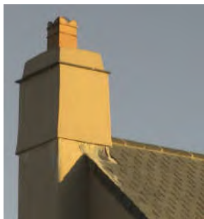
Gable end chimney, Camelford
