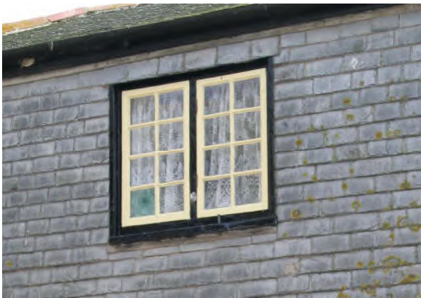
Hung slate scantling
