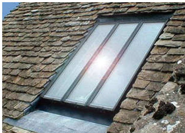
Conservation type of rooflight flush with the roof
