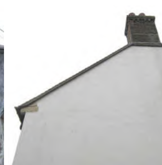
Simple Verges with wall finish taken up to underside of roof
