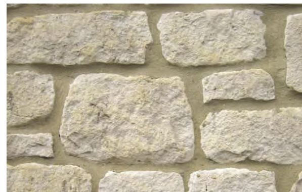
Stone and mortar joint sizes are well proportioned and colours are complementary.
