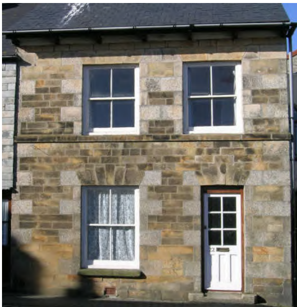
Sandstone wall with granite quoining
