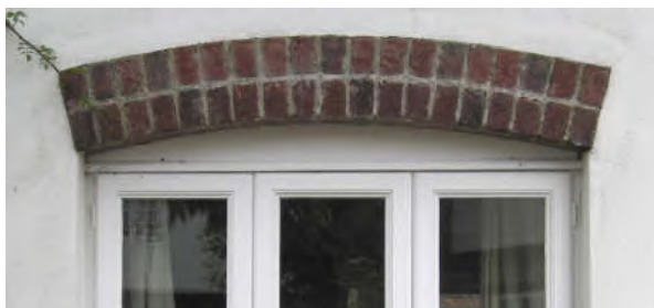
Segmented brick arch
