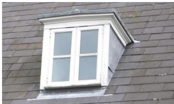
Good example of dormer window, lead details
